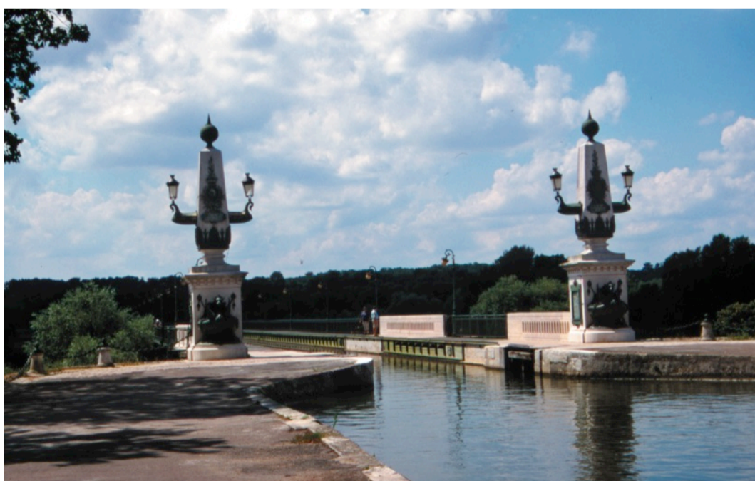
Three other aqueducts using cast iron: the first, at Longden-on-Tern; at Cosgrave, north of London; and at Briare, in France.
