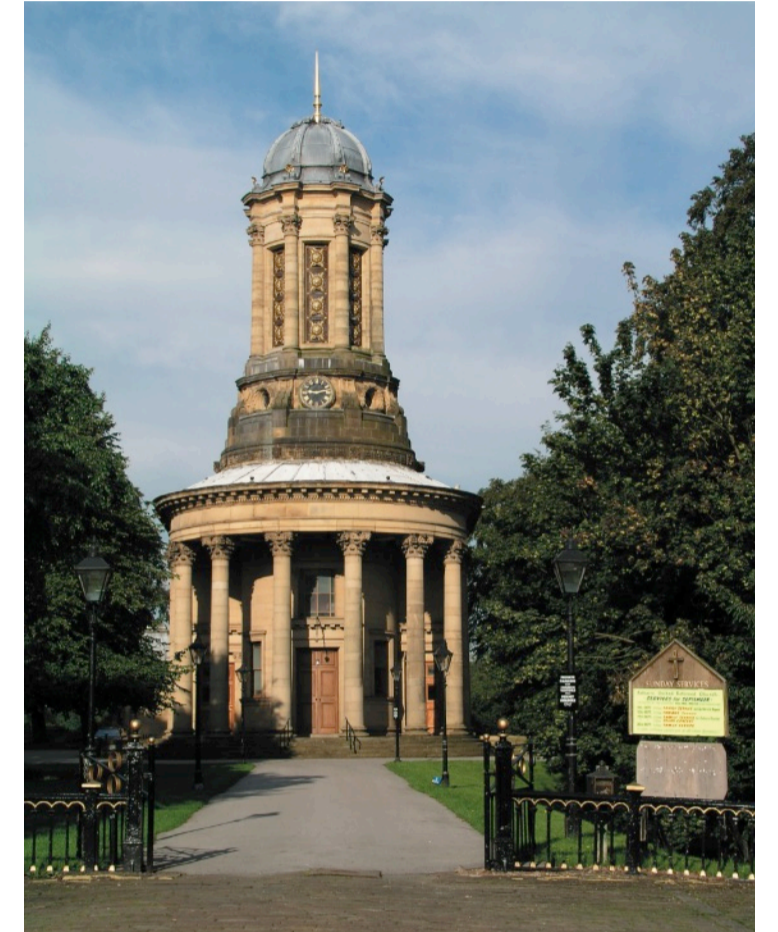
Several architectural influences can be seen in the Congregational Church, where Titus Salt would worship on Sundays.
